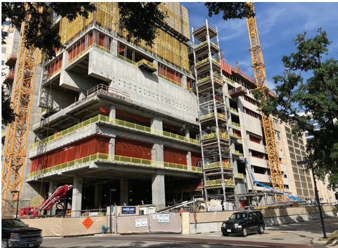
The Methodist Hospital System Centennial Tower project in the Texas Medical Center in Houston featured a 45 ft corner cantilever concrete transfer girder
